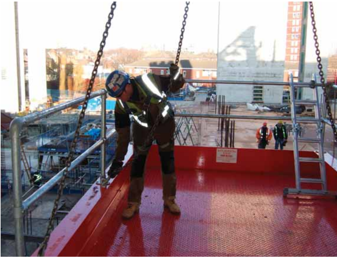
14 LOWER OFF ON THE CRANE UNTIL THE CHAINS COME LOOSE
