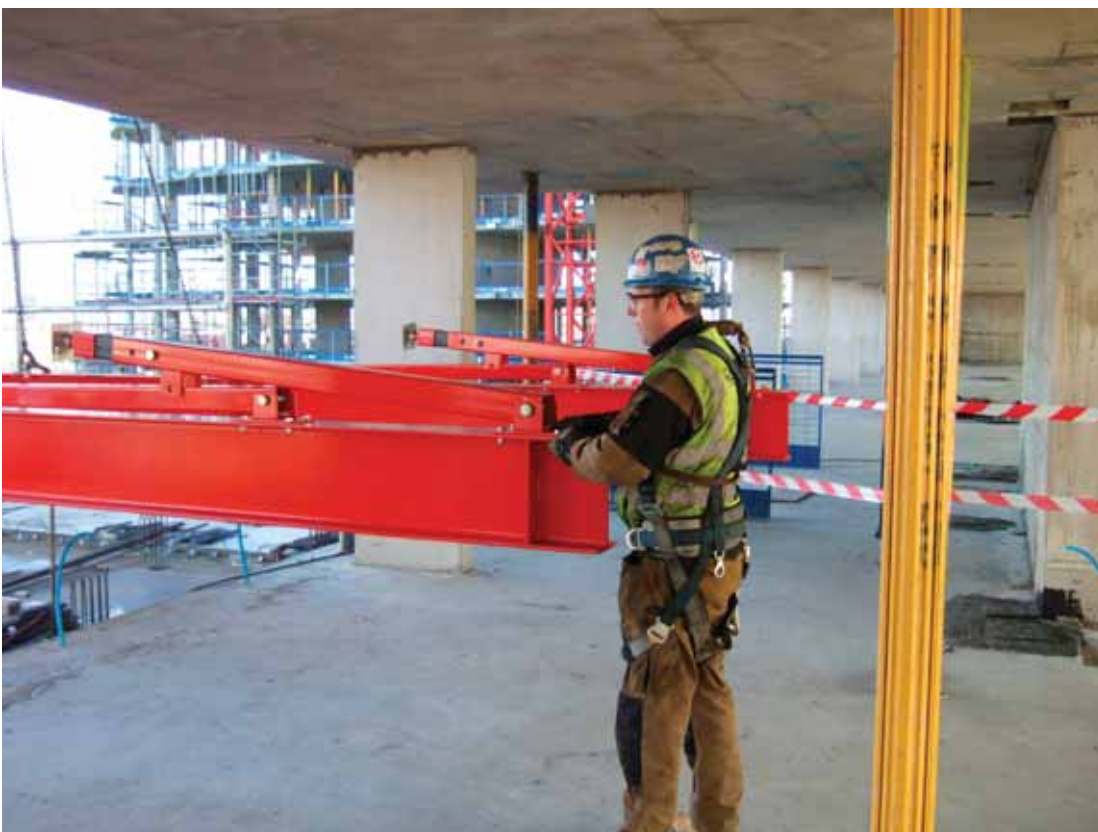
7 GUIDE THE PROP END OF THE PLATFORM INTO THE BUILDING
