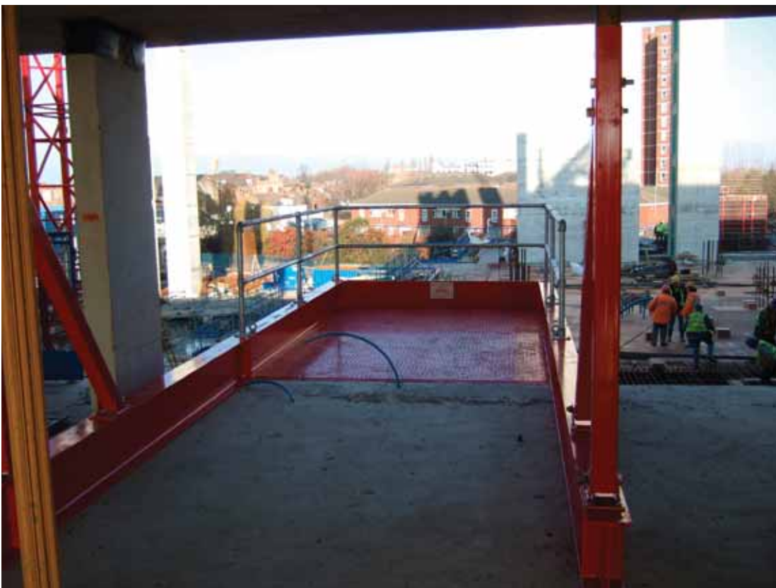
17 CARRY OUT FINAL INSPECTION ENSURING THE PROPS ARE TIGHT AND THE EASY-DECK PLATFORM IS NOW READY TO USE
