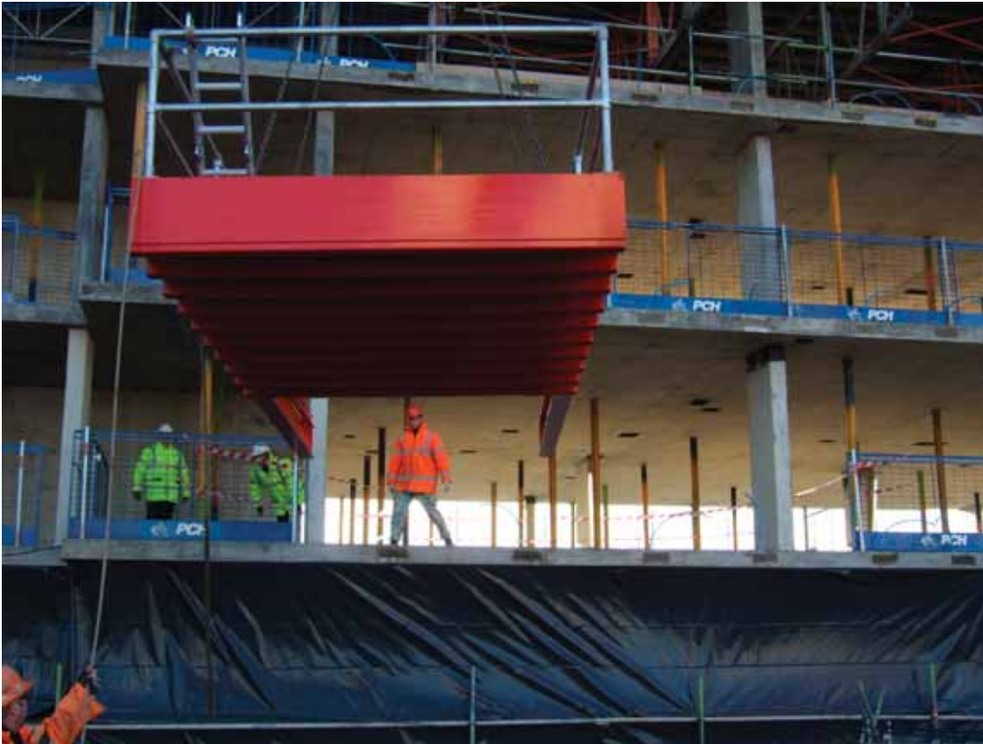
6 HOIST THE PLATFORM UP TO THE INSTALLATION POSITION USING THE TAG LINE TO CONTROL THE LIFT
