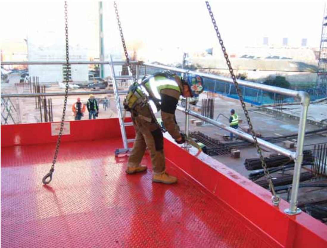
16 RELEASE THE CRANE CHAINS
